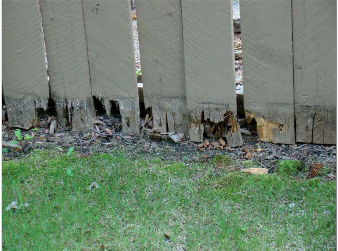
Photo 34: Wood fencing showing signs of advanced deterioration.
