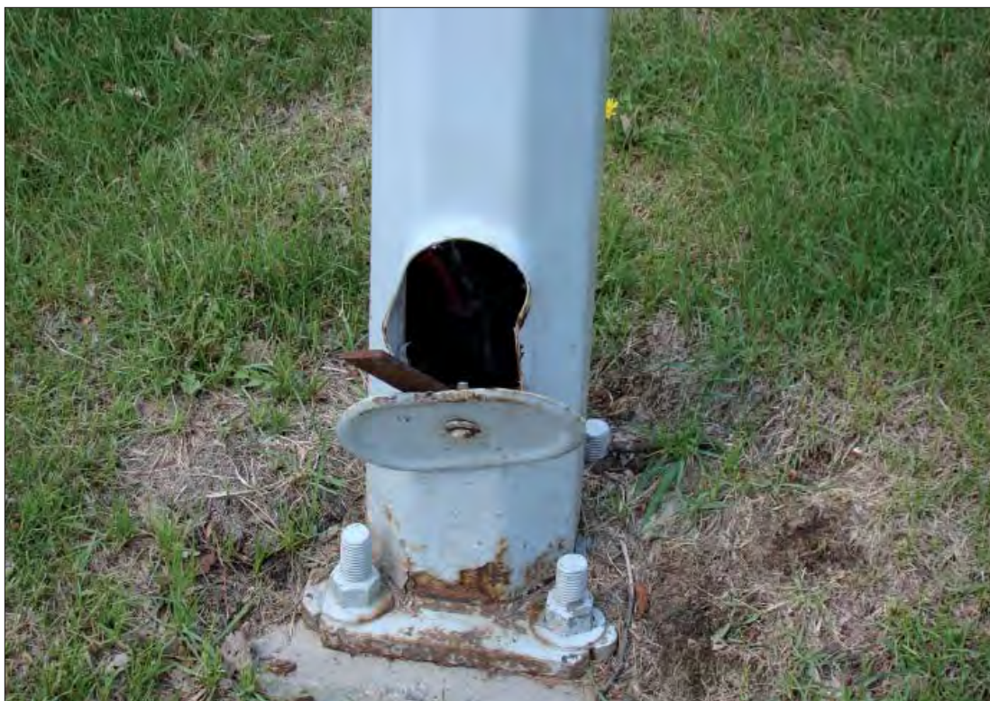
Photo 36: Walkway lighting with corrosion and exposed wires.
